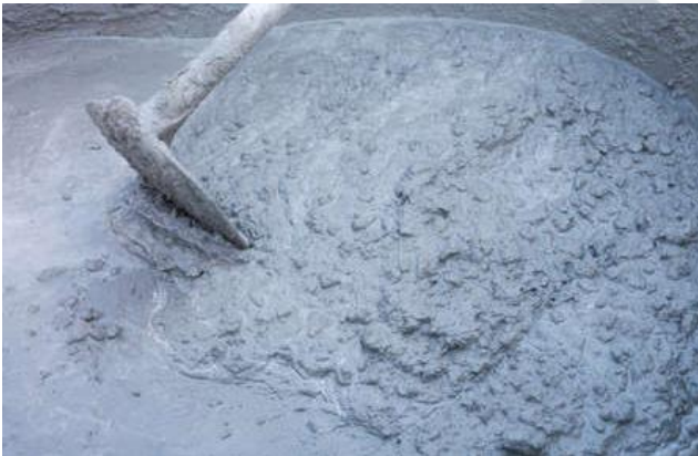
Figure 7. Mixing of Concrete Ingredients
